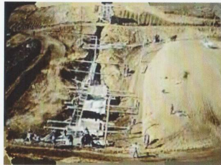
Setting forms for the concrete Corewall - 1911
