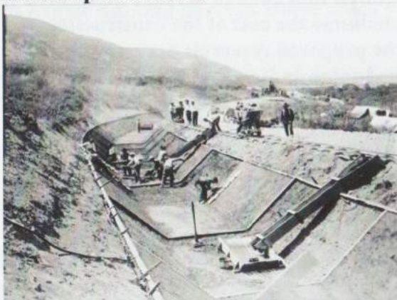
Setting forms for concrete in the Power Canal - 1908
