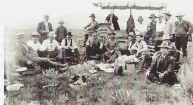
Workers at the Dam - 1911
