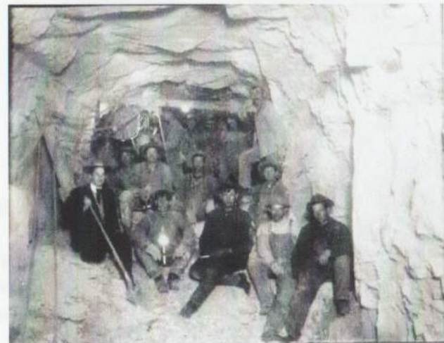
Heading crew inside the Tunnel - 1909
