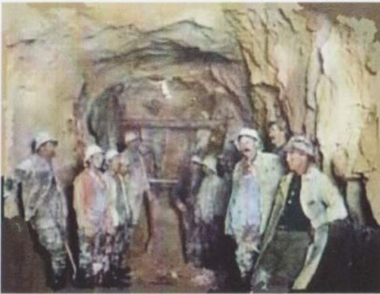
Workers inside the tunnel - 1909
