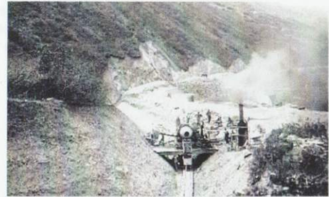
Lining the Power Canal with concrete - 1908
