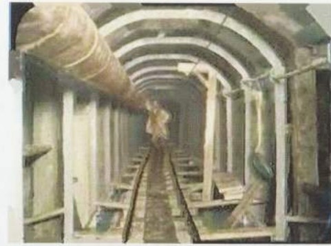
Worker inspecting the Tunnel ventilator duct - 1911
