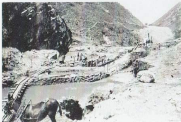
Power System to provide power for the compressed air drills-1908
