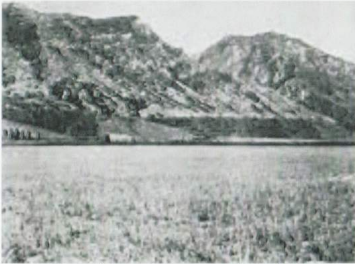
Dam site prior to construction - 1910
