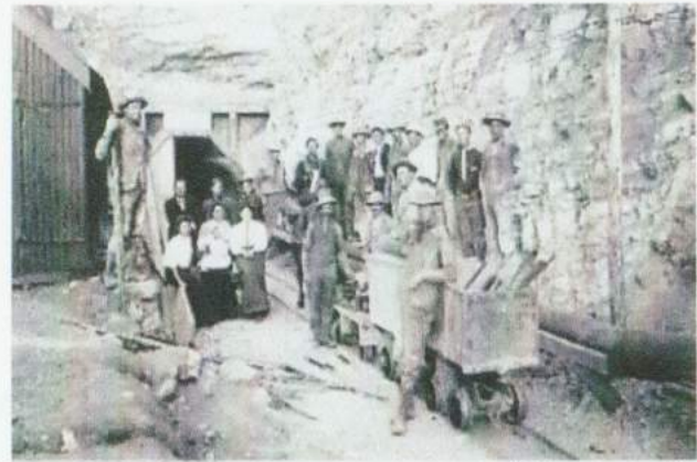
Workers at the West Portal entrance of the tunnel - 1909
