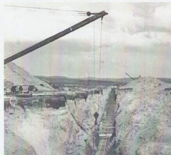
Setting forms for concrete in the Lateral - 1908
