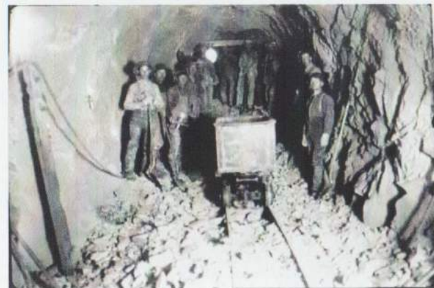
Heading crew loading a Muck car - 1909
