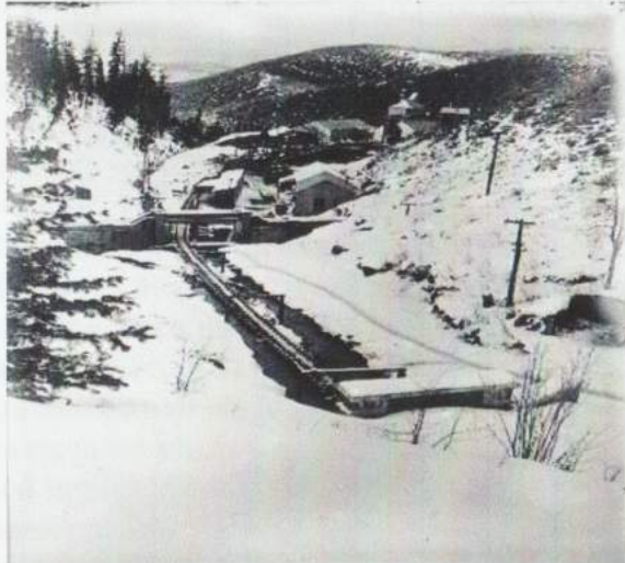
West Portal Weir & Machine Shop - 1908
