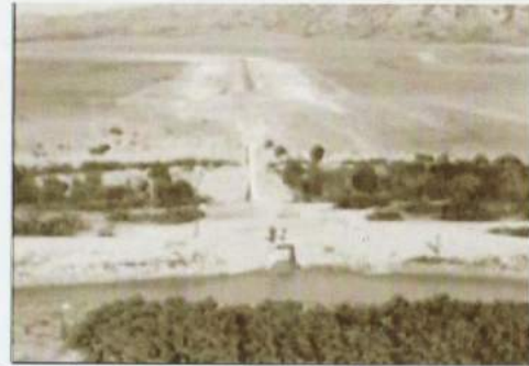
Completed section of the Lateral toward the tunnel entrance - 1911
