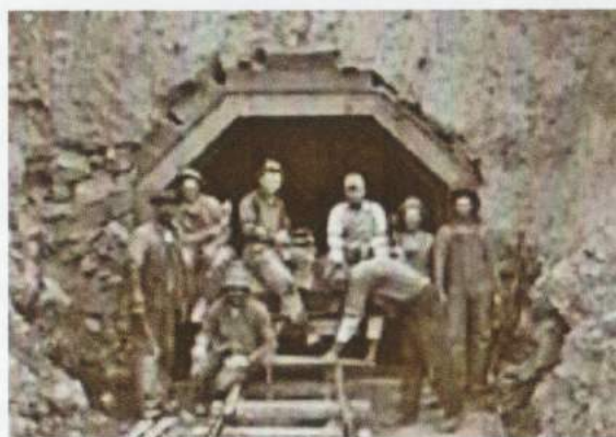
Workers at the East Portal entrance of the tunnel - 1909
