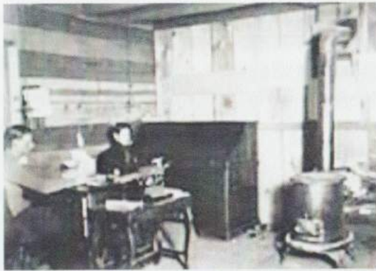
Strawberry Project Bureau of Reclamation office - 1906
