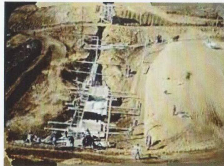
Setting forms for the concrete Corewall - 1911
