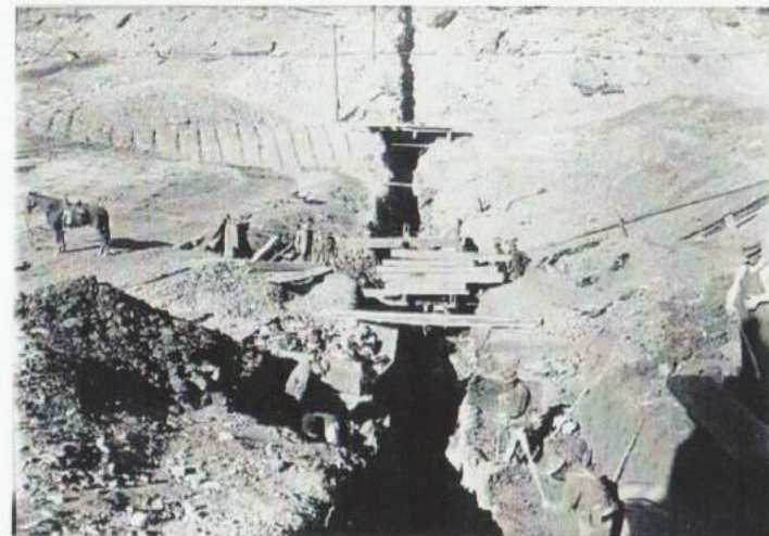
Digging the Corewall Trench - 1911
