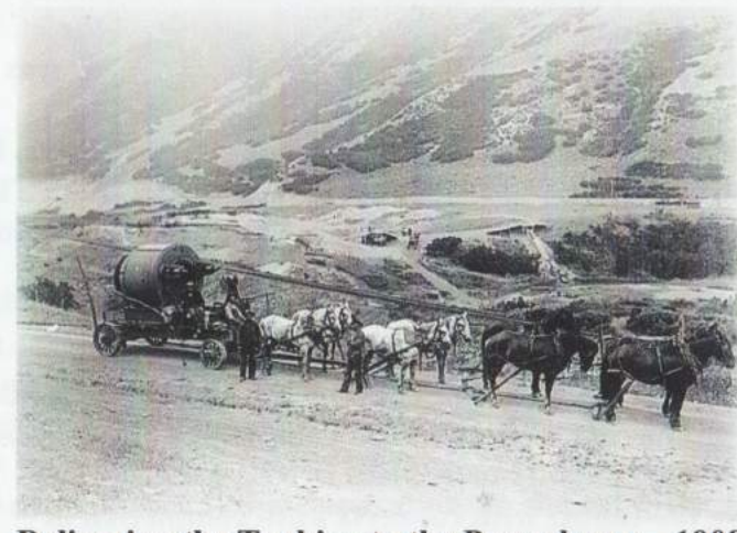
Delivering the Turbine to the Powerhouse - 1908
