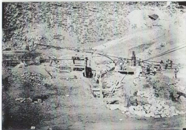
Dam Cutoff Trench - 1911
