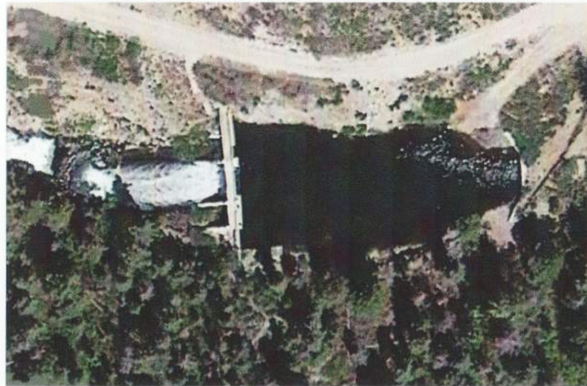
Sixth Water Aqueduct/Syar Tunnel discharge weir and spillway at the West Portal - ca. 1989
