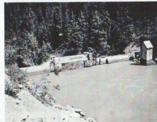
Tunnel discharge weir - 1951
