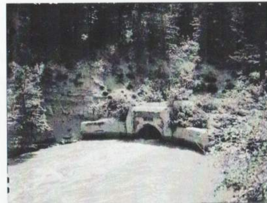
Tunnel discharge at the West Portal - 1951
