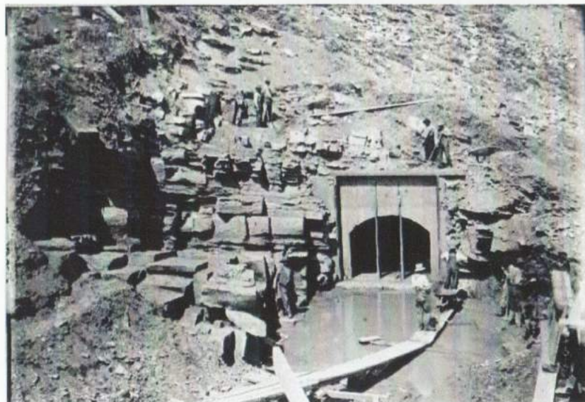
Tunnel intake at the East Portal - 1912
