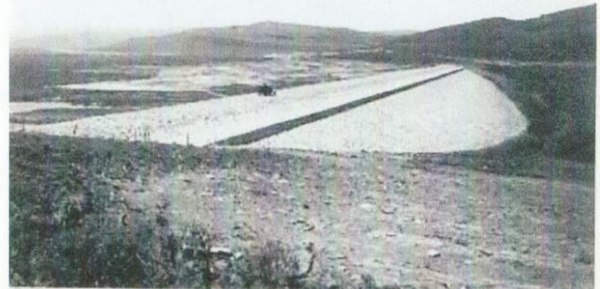
Hand-laid masonry on the upstream side of the completed Indian Creek Dike - 1912
