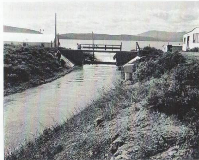
Indian Creek spillway - 1951
