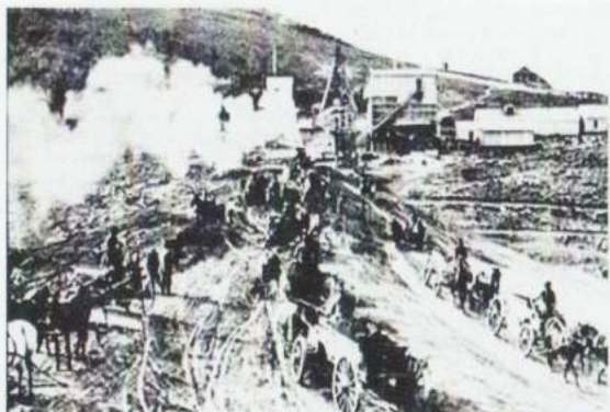
Rock crusher on the south side of the Dam - 1912
