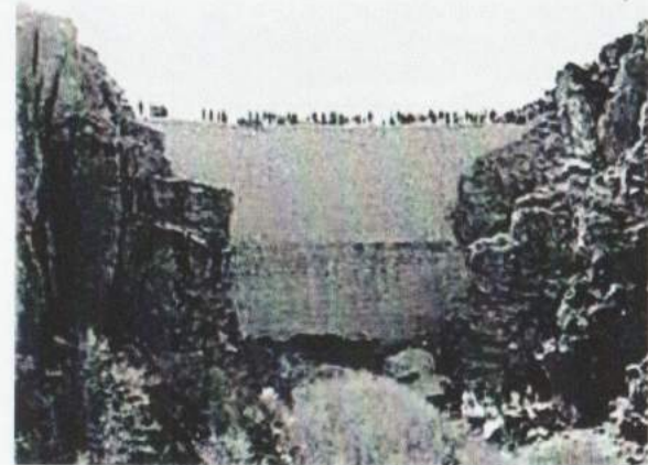
Back face of the dam - 1913
