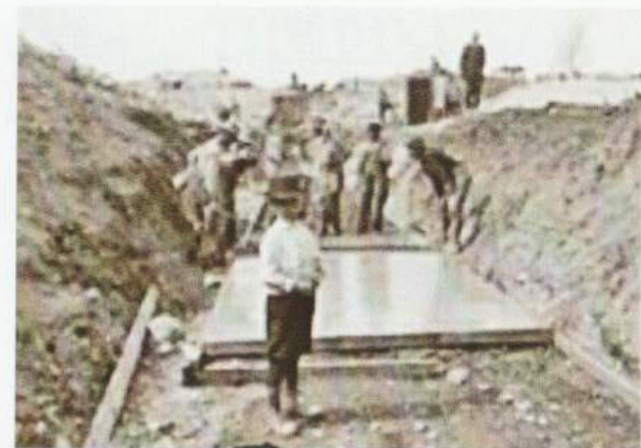
Workers laying out ground slabs for the concrete culvert - 1913
