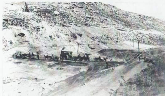
Steam roller with leveler on the dam - 1912
