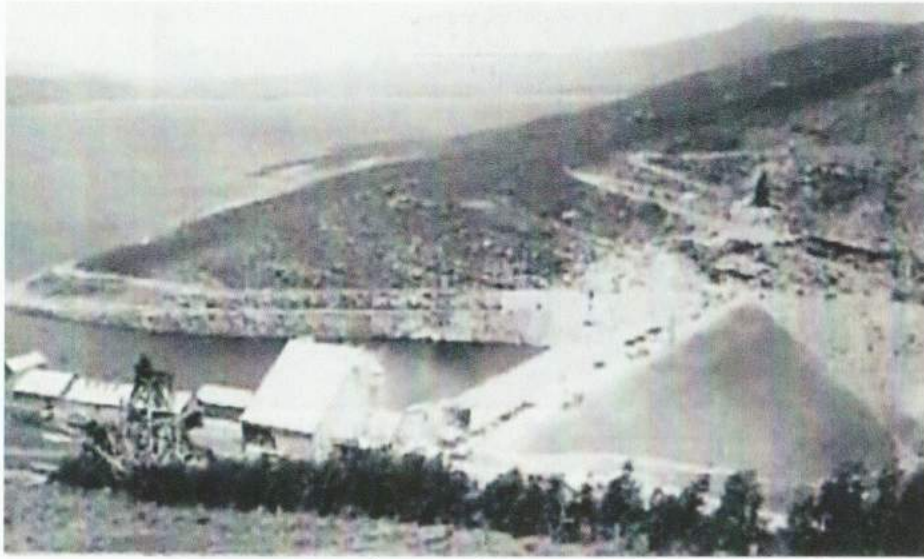
Dam construction nearing completion - 1913
