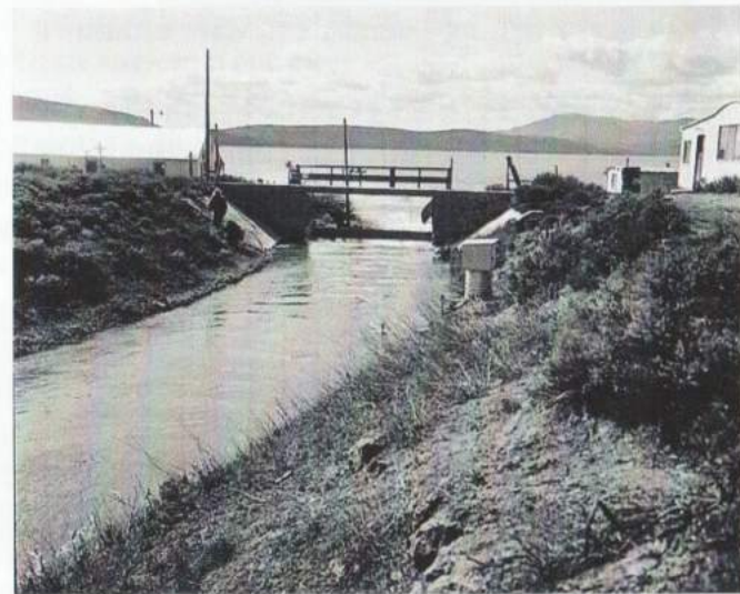
Indian Creek spillway - 1951
