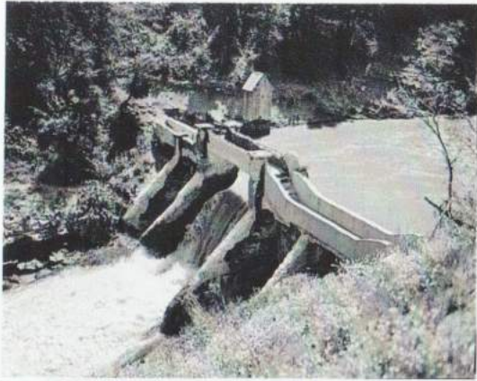
Tunnel discharge weir and spillway - 1951
